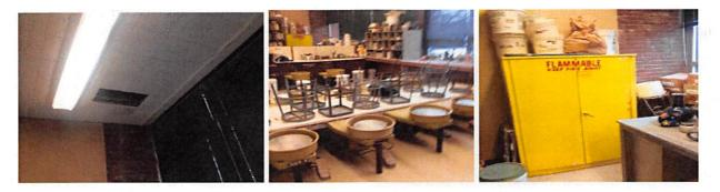
Pictured ceiling tile needs to be replaced. Good housekeeping noted around pottery wheeling. Reposition items stored on top of flammable storage cabinet to a lower level.
