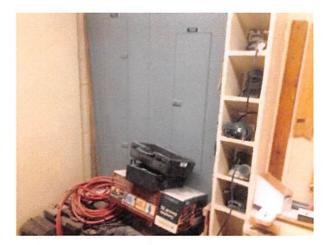
OSHA 29 CFR 1910.303- Access-3 foot access required to all electrical panels or disconnect switches. Rearrange tiems so there is direct access to the electrical panels.
