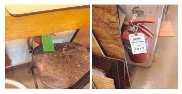
OSHA 1910.157(c)(1) The employer shall provide portable fire extinguishers and shall mount, locate and identify them so that they are readily accessible to employees. Both pictured extinguishers have expired tags. Relocate the pictured extinguisher on the left to an area more accessible.
