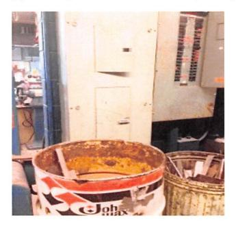
OSHA 29 CFR 1910.303- Access-3 foot access required to all electrical panels or disconnect switches. Rearrange tiems so there is direct access to the electrical panels.
