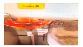
OSHA 29CFR 1910.151 & ANSI Z358.1-2004 Regulations- Plumbed emergency fixtures should be tested on a weekly basis long enough to flush the line of sediment. All eyewash and showers shall be tagged to show inspection dates- weekly and annual inspections shall be documented.
