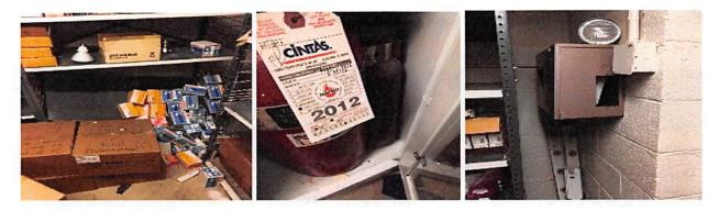
Pictured shelf is in need of repair. Fire extinguisher expired. The pictured emergency lighting shall be tested for proper operation.
