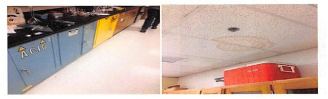
Pictured acid cabinets in good condition, no excess corrosion noted. Pictured ceiling tile shall be replaced.
