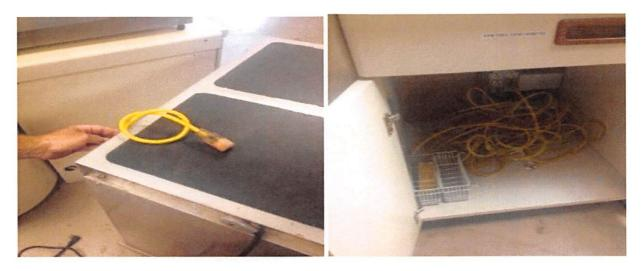
Extension cords shall not be used as a permanent means of electricity. Efforts shall be made to determine the power source and change it to an outlet. The pictured extension cord is used for the warmer. Efforts shall be made to see if the warmer can be hooked up to a permanent power source. If extension cord is to be used, storage of the cord needs to be improved and wrapped in a manner to prevent any frays or damage to the cord.
