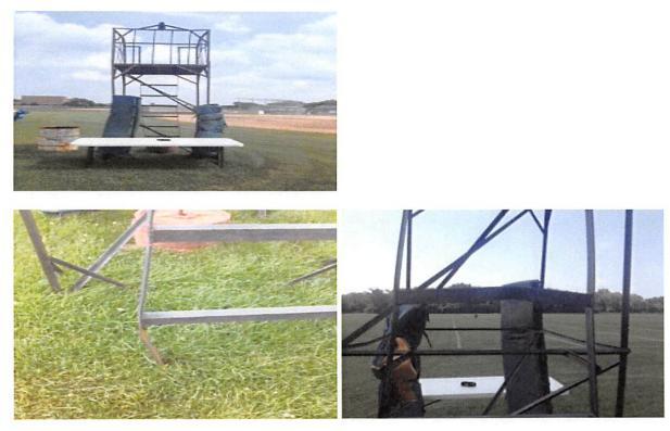
It is recommended that the pictured filming tower is removed from use. The ladder access to the platform has several un-level sections. Due to areas of bent metal surrounding the legs of the structure its stability may have been compromised.
