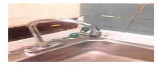
OSHA 29CFR 1910.151 & ANSI Z358.1-2004 Regulations- Plumbed emergency fixtures should be tested on a weekly basis long enough to flush the line of sediment. All eyewash and showers shall be tagged to show inspection dates- weekly and annual inspections shall be documented. Check the water pressure of the pictured eyewash. Upon activation, pressure was low.
