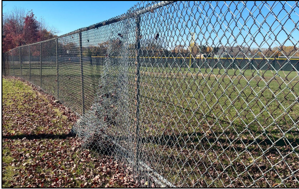
Image 3 - Existing Perimeter Fencing Along Sherman (GBN)
