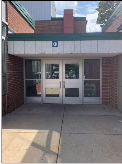
Image 5 - GBN Wood Soffit Repair
