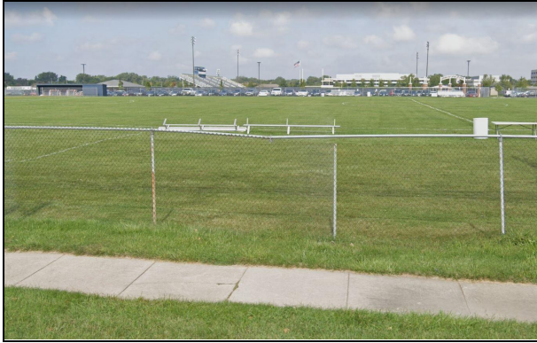
Image 1 - Existing Perimeter Fencing Along Lake (GBS)
