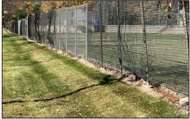
Image 2 - Existing Perimeter Fencing Along Sherman (GBN)
