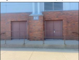
The aluminum doors are typically part of an overall glazing system and are used in places to provide architectural detail, primarily at the main entrances. Hollow metal doors are usually found at utility entrances and doors going into specific building areas, such as music rooms, gymnasiums, natatoriums, fieldhouses, scene shops, automotive classrooms, etc.
