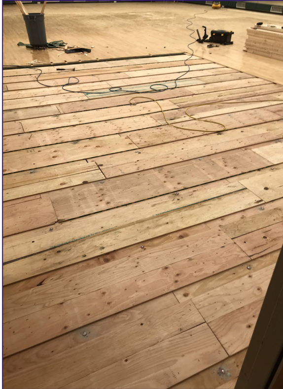
Sub-flooring Installation
