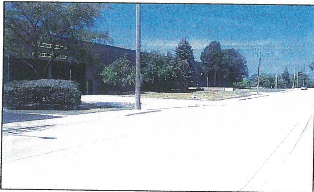
VIEW OF SUBJECT'S EAST ELEVATION FROM HUEHL ROAD FACING NORTHWEST
